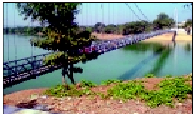
Dhableswar Bridge constructed under RIDF in Orissa
