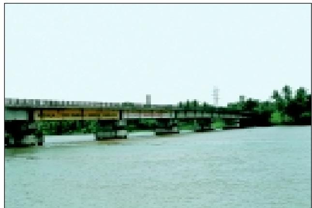
Bridge constructed under RIDF in Kerala
