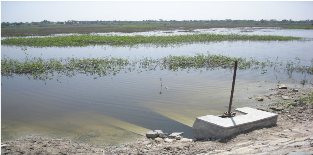
Photo 9: Tank Improved Sluice Control, Karnataka
