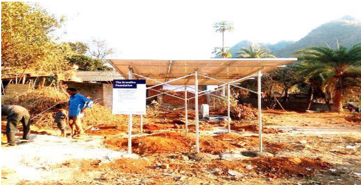
Photo 2: Solar Tube well
