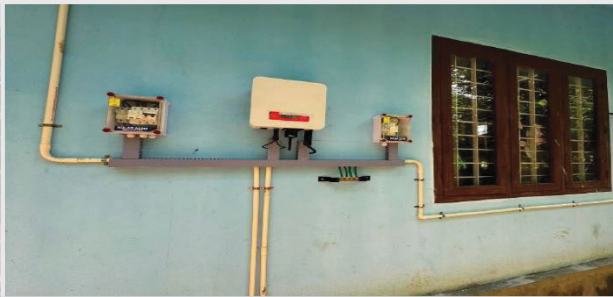
A 2-kilowatt grid-connected solar photovoltaic system; Anganwadi no. 129, Kerala.
