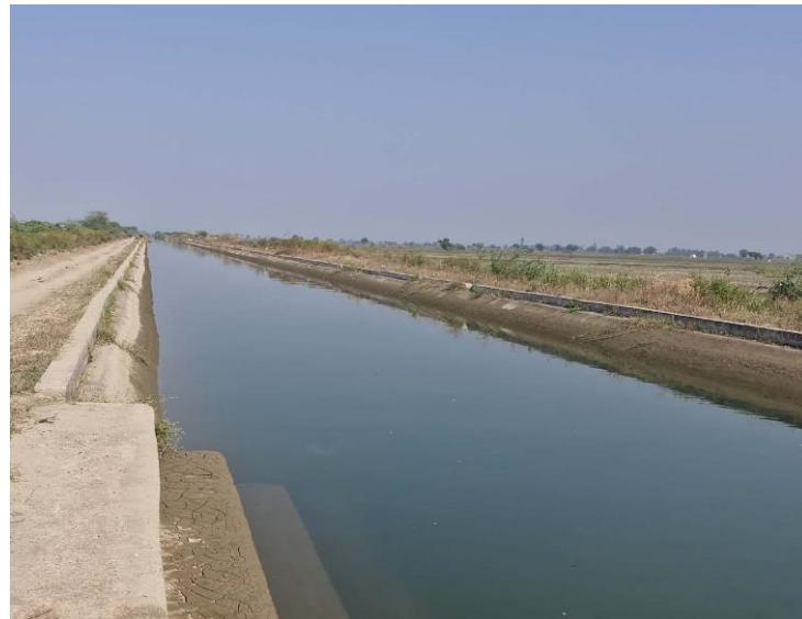
For decades, farmers relied on a 30.88kilometer Barod subBranch unlined earthen canal that carried water from Dabar Branch which is offtaking from Right Main Canal of Chambal Irrigation Network. While essential for irrigation, the unlined canal suffered heavy seepage, silting, and vegetation growth. As a result, over 40% of the water was lost before it could reach the fields. Crop yields declined, and many farmers began shifting to less water intensive , lower remunerative crops.
