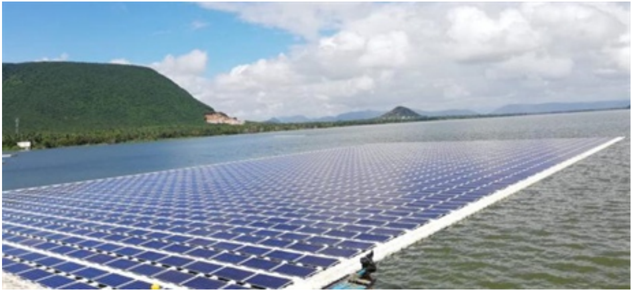
Meghadri Gedda Reservoir: Floating Solar Plant, Vishakhapatnam
