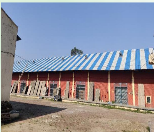
Replacement of old Asbestos Sheet Roofing of godowns with Galvanized Iron profile sheet
