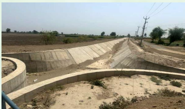
Cement Concrete Lining of Bahadurke Distribution System
