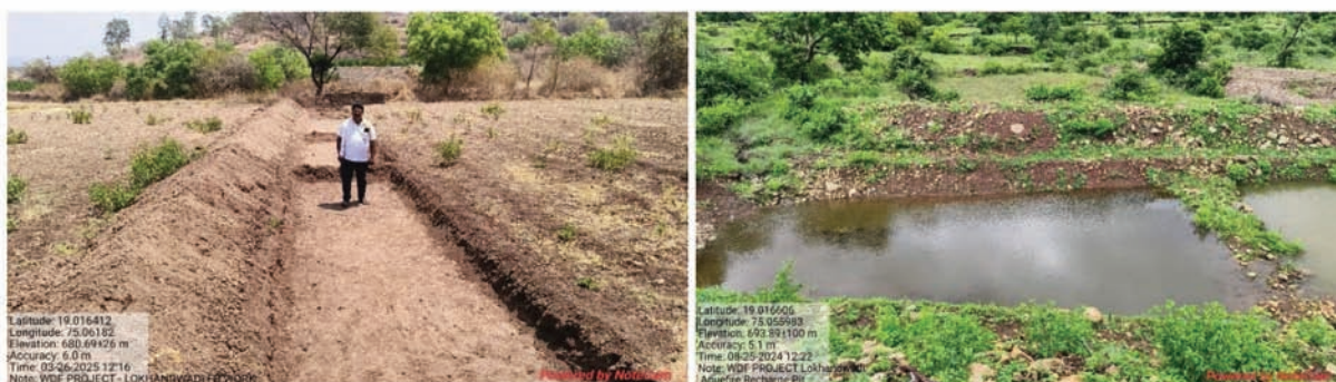
Farm Bund and Aquifer Recharge Pits in Lokhandwadi watershed project of Beed district
