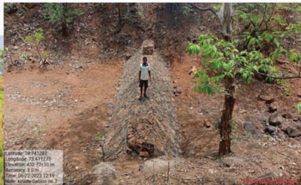
Gabion structure under Udhale springshed project of Palghar district
