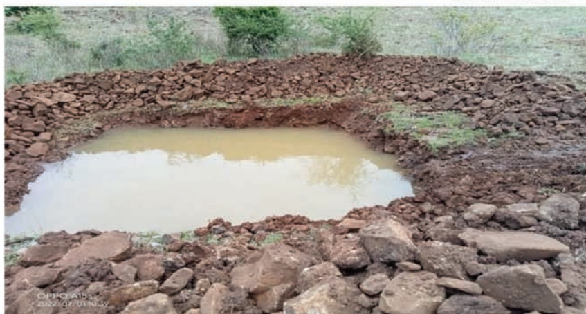
Recharge pits constructed at Ghodaj KfW-SEWOH-III project of Nanded district
