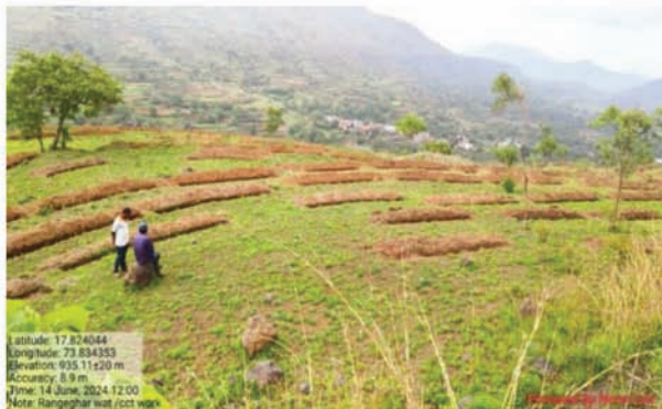
Continuous Contour Trenches in Rangeghar springshed project of Satara district
