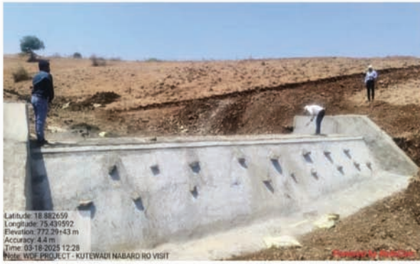
Check dam built in Kutewadi watershed project, Beed district ; Cement Nala Bund at Athnur Project of Latur district
