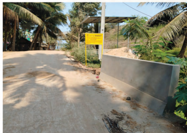
Bridging Communities: Culvert Constructed with NABARD RIPF Assistance
