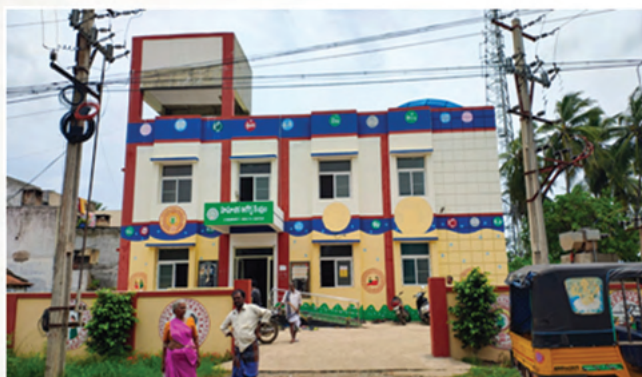
Community Health Center at Alamuru Mandal constructed under RIDF
