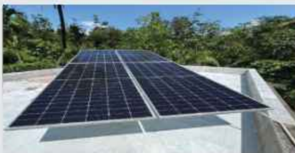
A 2-kilowatt grid-connected solar photovoltaic system; Anganwadi no. 129, Kerala.
